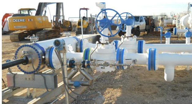
Figure 15 – Inferred Prover Installation
